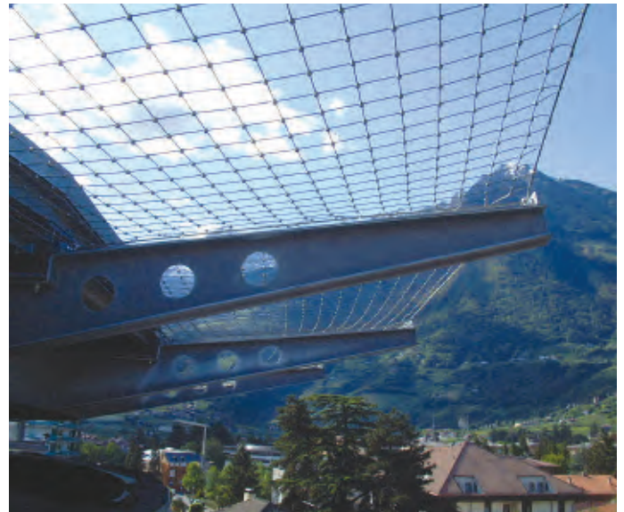
Dralo® used to secure the edges of a helicopter landing pad at a hospital in Meran.
