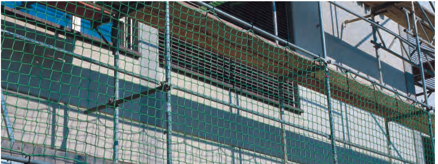
Brick guardrail net, mesh size 100 mm.
