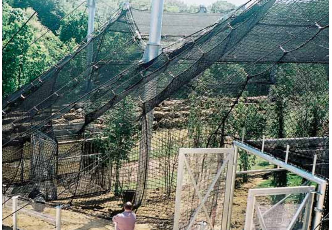
Installation by Huck-Torimex, Mondo Verde bird park in Landgraaf, the Netherlands.
